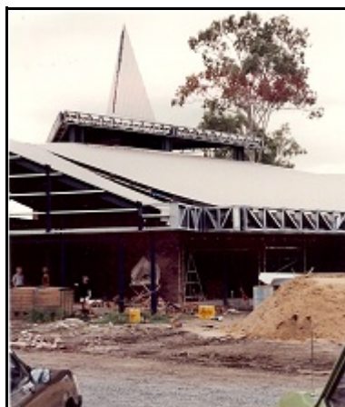
The multi-purpose building in Bray Park under construction.
