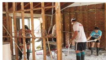
Many homes had to be stripped back to bear stud work.
